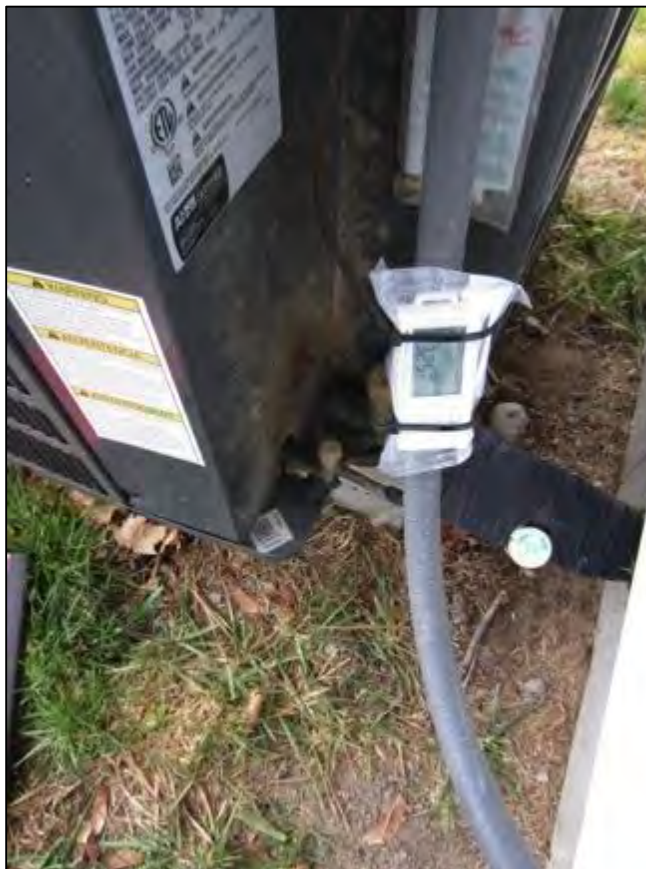
Figure 29. Motor Logger on Electric Conduit to Condenser
