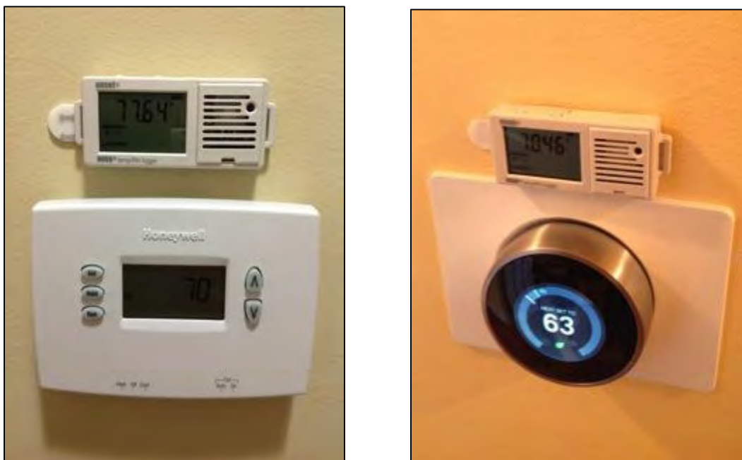
Figure 27. Thermostat Logger Installed Near Programmable (left) and Nest (right) Thermostats
