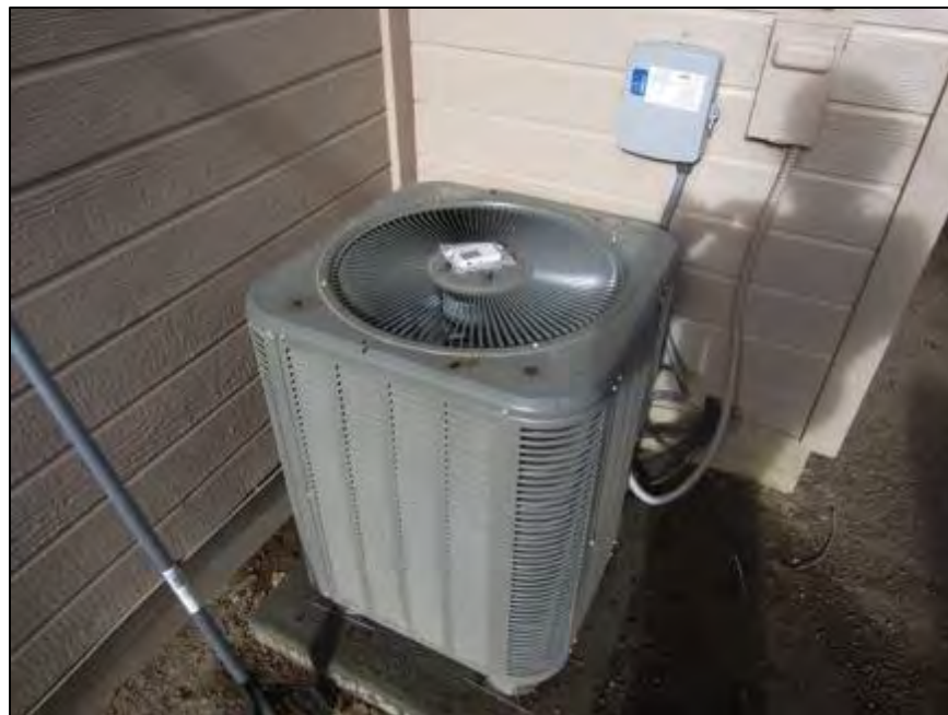
Figure 28. Motor Logger on Condenser
