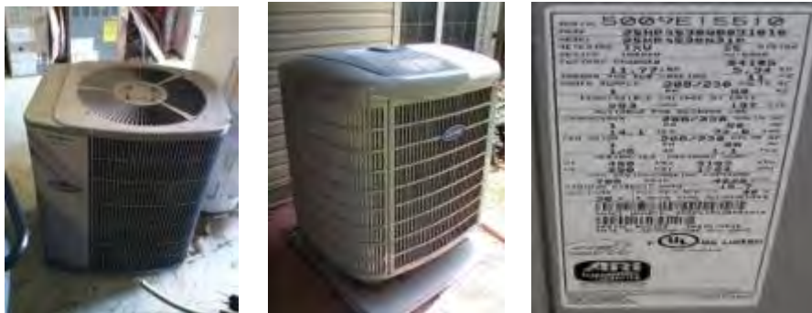
Figure 26. (Left to right): Standard 2.5-Ton Carrier Air Conditioner, Standard 2.5-Ton Carrier Heat Pump, Nameplate of Heat Pump
