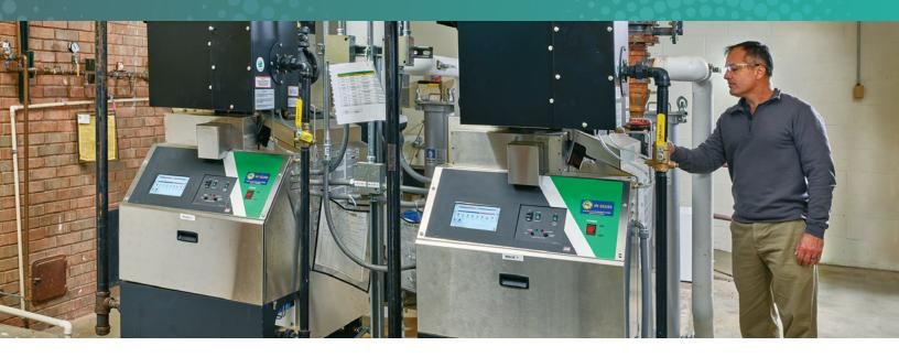
A boiler tune-up can improve boiler efficiency by more than 5%. It is recommended that a tune-up be performed annually by a qualified technician as part of a regular maintenance schedule. Besides saving energy and lowering operating costs, a boiler tune-up helps to:
